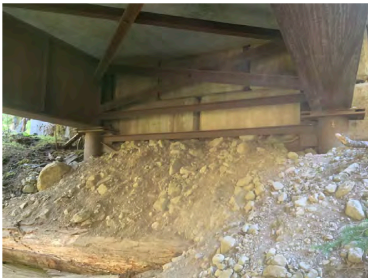
Right Bank Abutment when facing downstream
