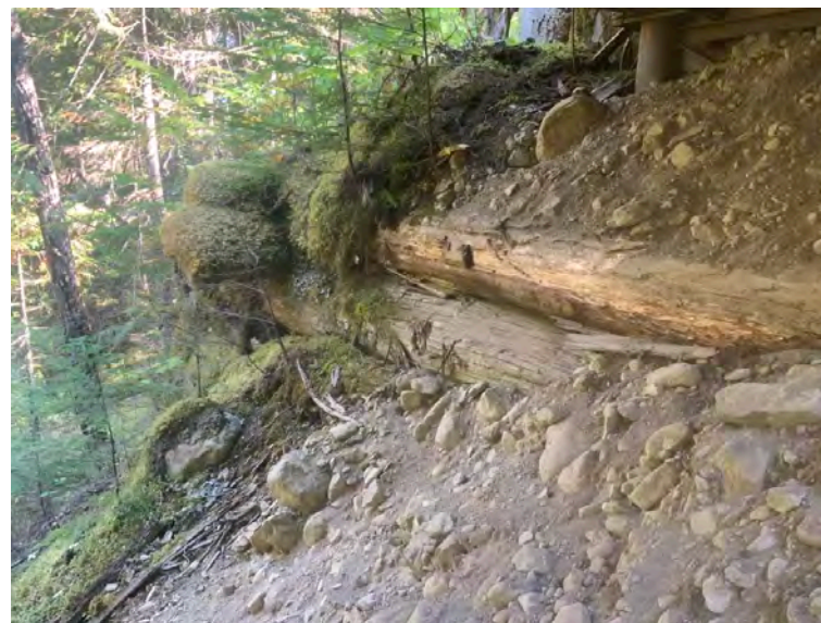
Right Bank Abutment when facing downstream
