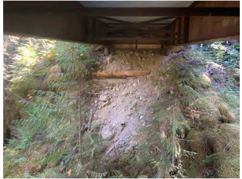
Right Bank Abutment when facing downstream
