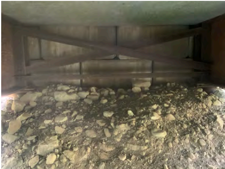
Left Bank Abutment when facing downstream
