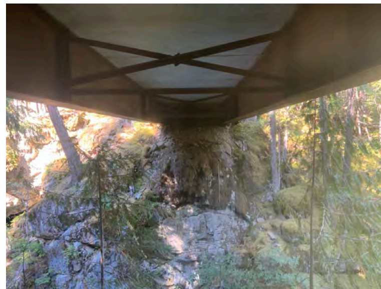
Left Bank Abutment when facing downstream
