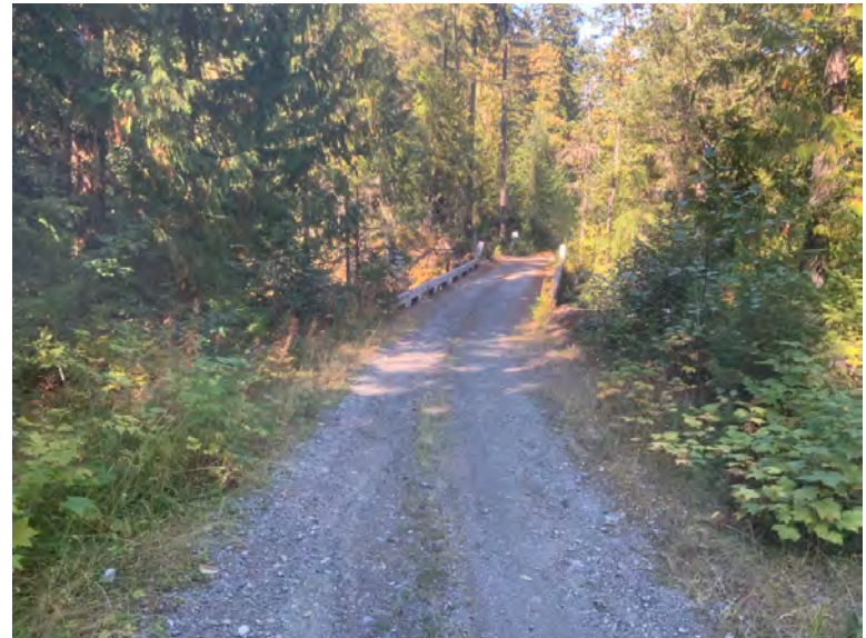
Approach from Right Bank when facing downstream
